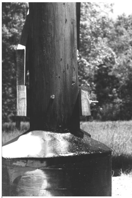
**Photo 33.** Tower pole and concrete collar connection. Note taper of concrete. *Photo courtesy of Mr. Tibor Latincsics.*
