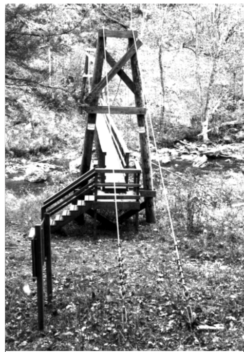
Photo 11. Inclined towers of the Jackson River Bridge. Photo Courtesy of Mr. Tibor Latincsics.
