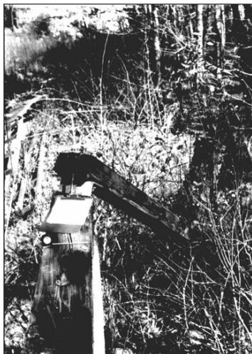
**Photo 53.** The timber towers were sheared at the base by floodwater driven debris. *Photo courtesy of Mr. Tibor Latincics.*
