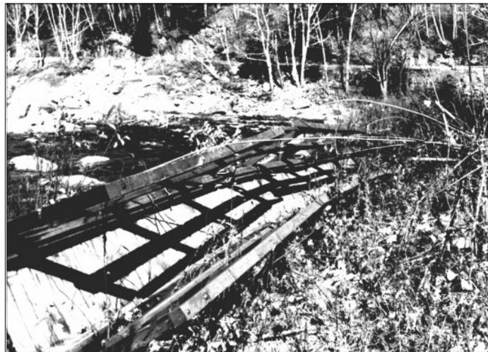
**Photo 54.** Hastings Bridge walkway remains flung downstream. *Photo courtesy of Mr. Tibor Latincics.*
