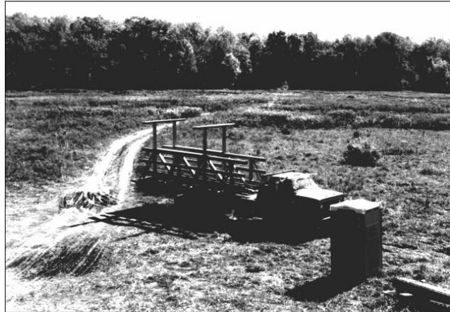
**Photo 50.** Fabricated bridge sections were trucked to the site by the NJ Forest Fire Service. *Photo courtesy of Mr. Tibor Latincsics.*
