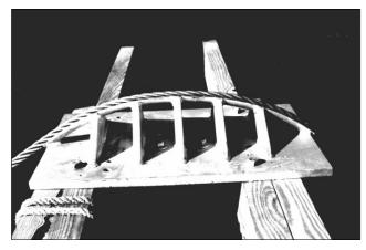
**Photo 51.** West tower - north pole cable saddle. *Photo courtesy of Mr. Tibor Latincsics.*
