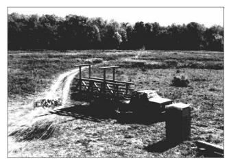
**Photo 50.** Fabricated bridge sections were trucked to the site by the NJ Forest Fire Service. *Photo courtesy of Mr. Tibor Latinosics*.
