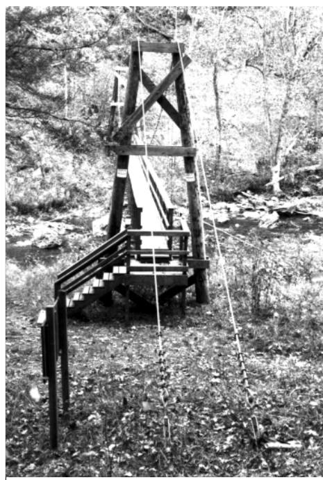
Photo 11. Inclined towers of the Jackson River Bridge. Photo Courtesy of Mr. Tibor Latincics.
