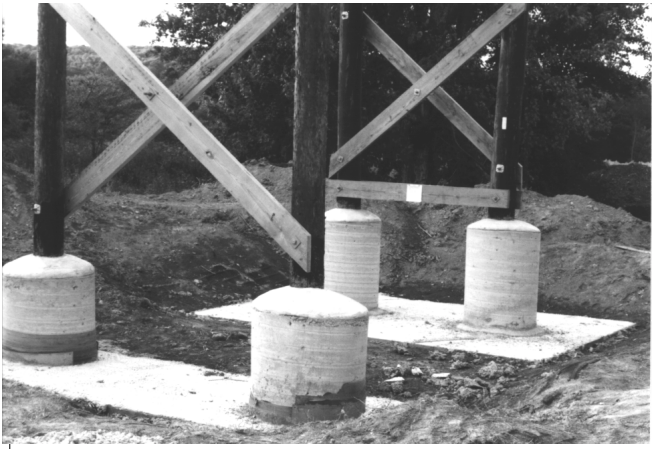
Photo 31. Foundation after concrete had set, but before backfill. Photo courtesy of Mr. Tibor Latincsics.
